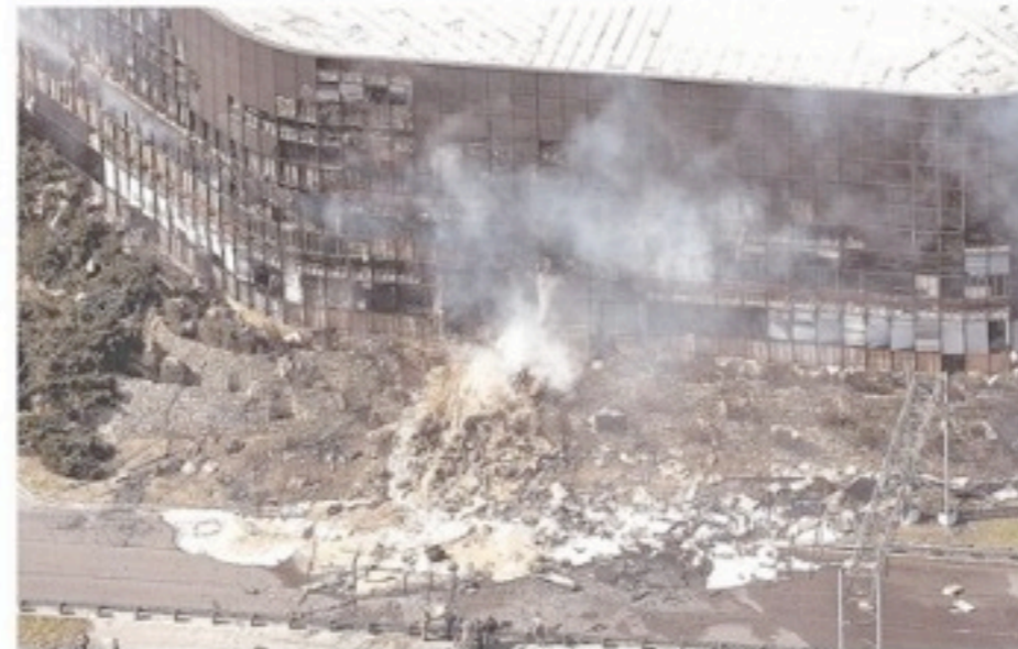
Smoke billows from a seven-story building in Austin, Texas, after a man who once lived in Harrisburg crashed a plane into the structure, which houses an IRS office. BELOW: Firefighters work on the second floor. Remnants of the plane are at bottom.
